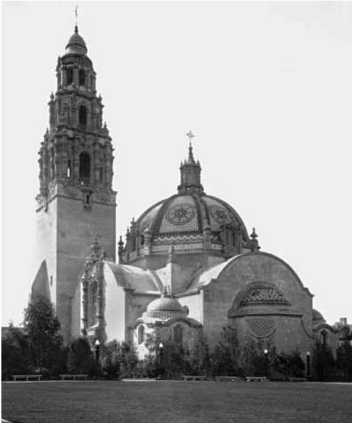
California building completed in 1914. ©SDHC #852.
