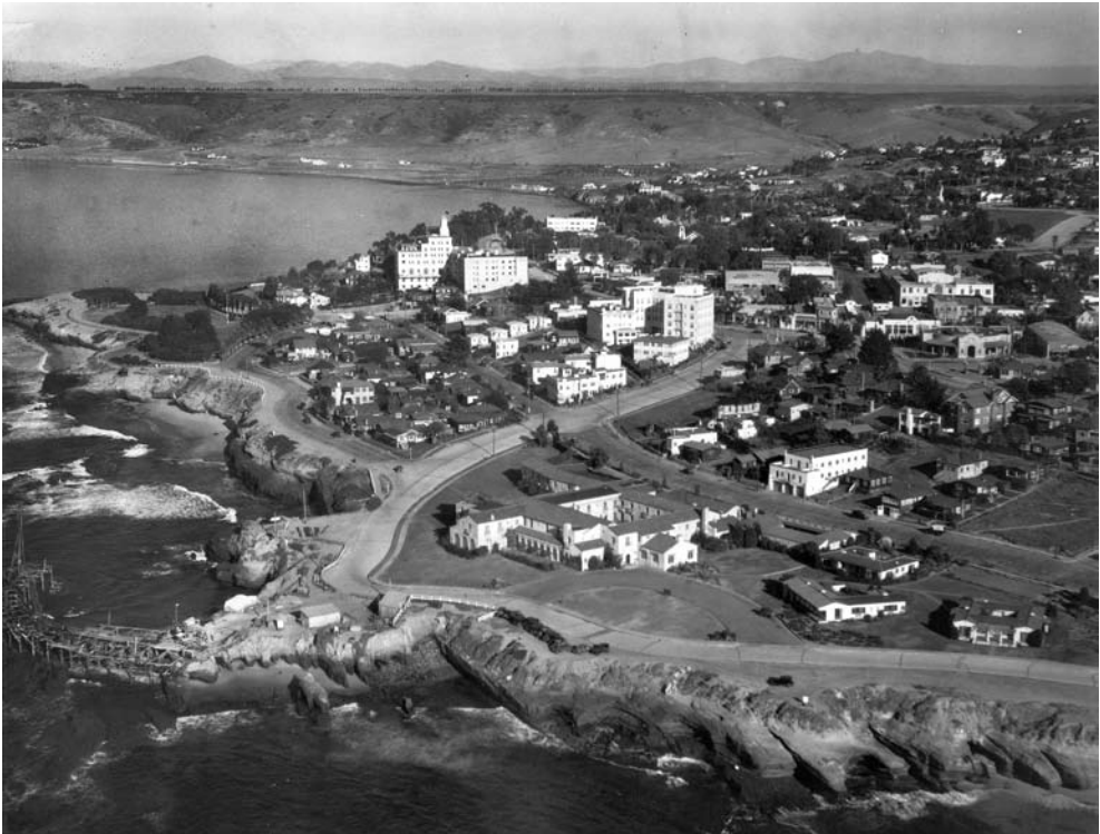
View of La Jolla showing the Children's Pool under construction, ca. 1931. ©SDHS, #90:18138-444-
